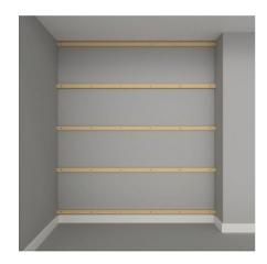
Securely drill and fix five battens (45mm x 45mm) to the wall, evenly spaced. You have the option of installing mineral wool between the battens to improve insulation and increase sound absorption.
