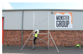
Always climb up the inside of the ladders and carefully manoeuvre through the trapdoor.
